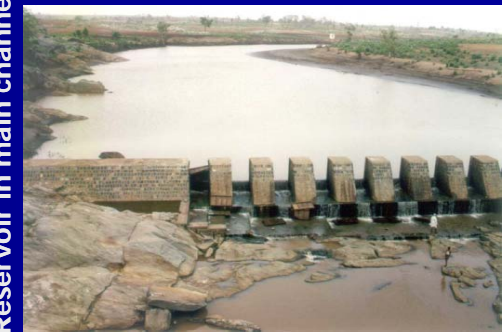
Reservoir in main channel
