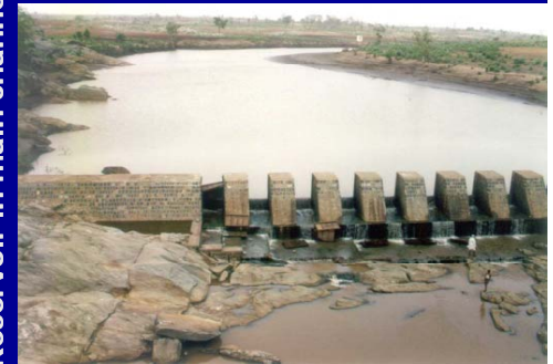
Reservoir in main channel
