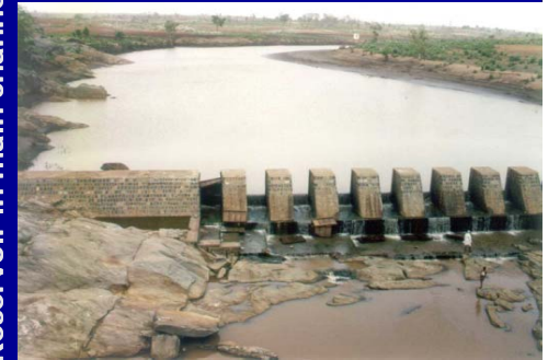
Reservoir in main channel
